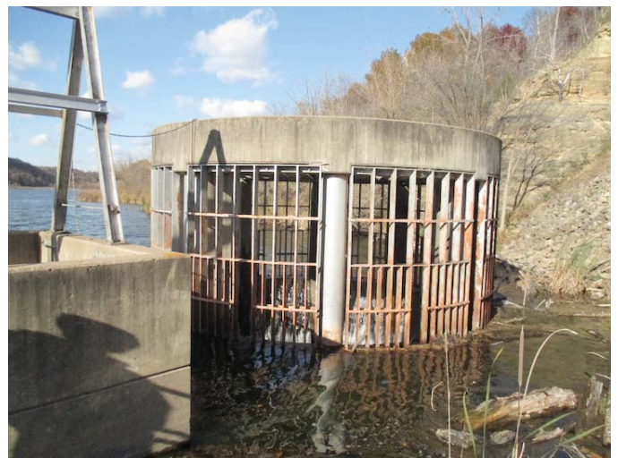
The dam's intake structure.
