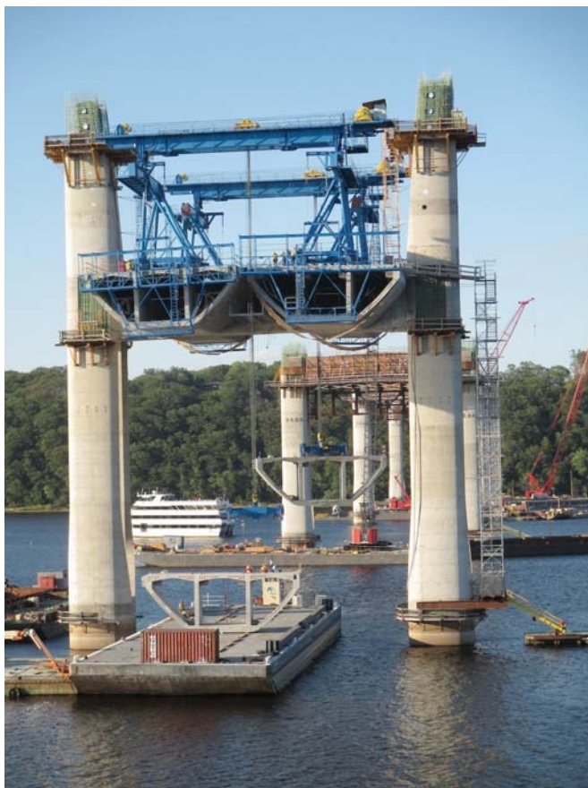
Lifting a segment to the pier table.
