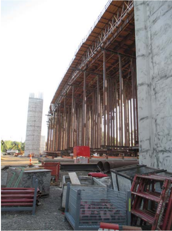
The cast-in-place approach spans with a few pieces of rebar.
