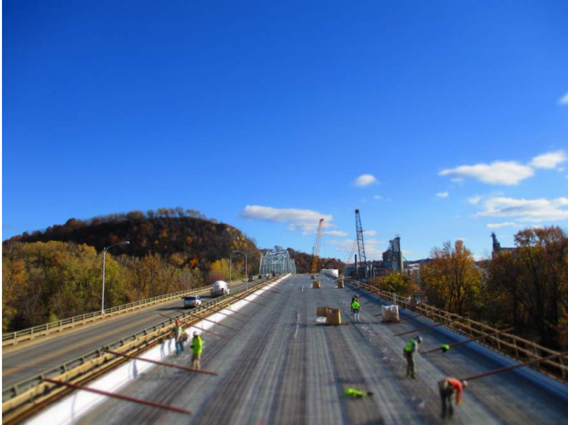
Steel workers tying rebar to prepare for an upcoming deck pour
