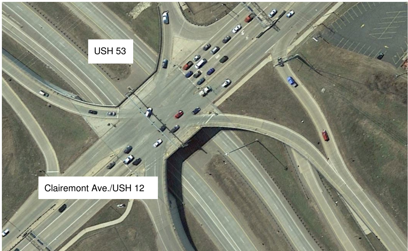
The final constructed Single Point Urban Interchange in Eau Claire (Source: Google Earth).
