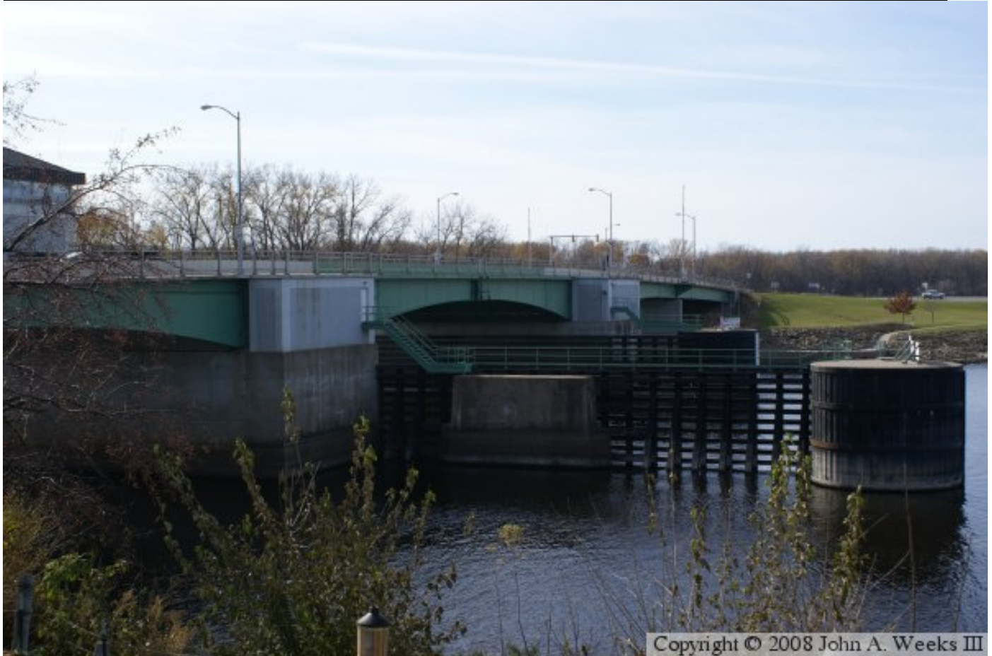
The Point Douglas Drawbridge, looking southwest into Minnesota. Notice the piers of the original lift bridge.
