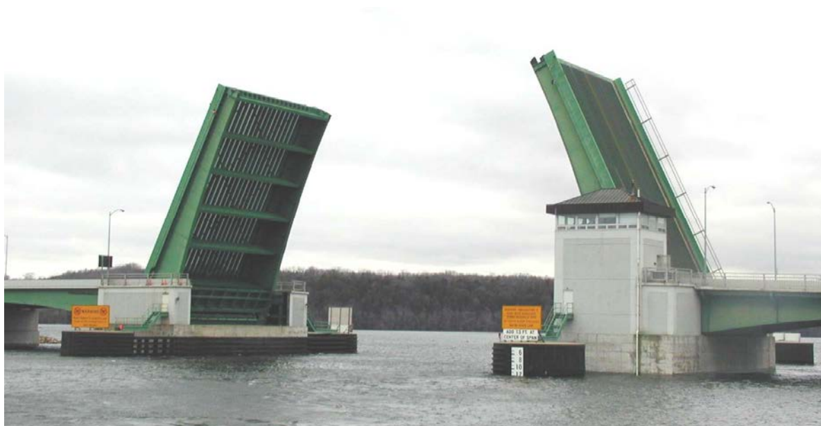
The Point Douglas Drawbridge, open and ready for boat passage. (Source: WisDOT)
