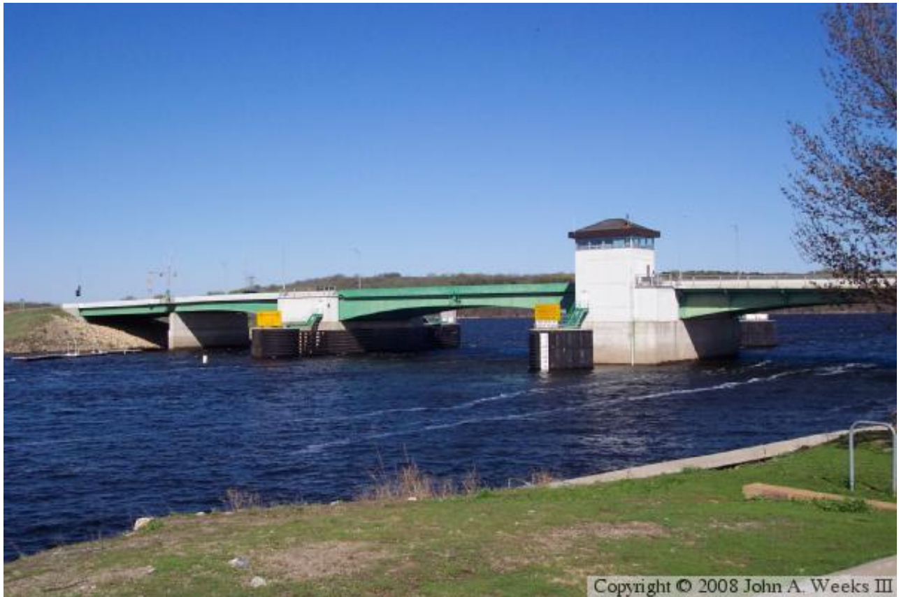
The Point Douglas Drawbridge, looking north.
